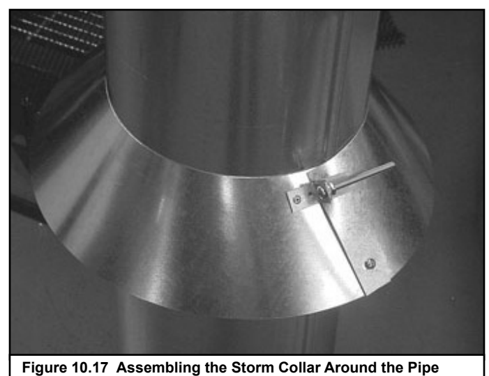
Figure 10.16 Assembling the Storm Collar
